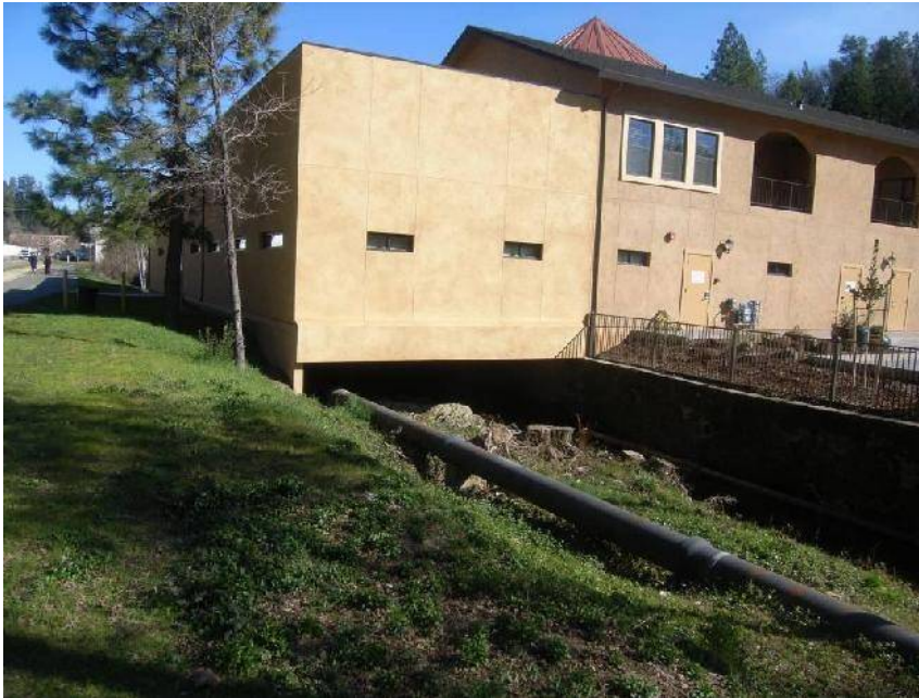
Photograph 1: Building near Locust Avenue
