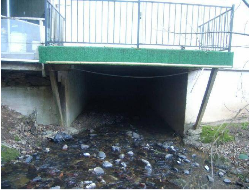
Photograph 3: Building Adjacent to Broadway near Smith Flat Road
