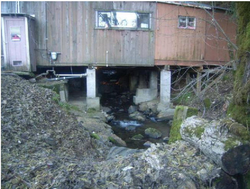
Photograph 2: Building Adjacent to Broadway near Smith Flat Road
